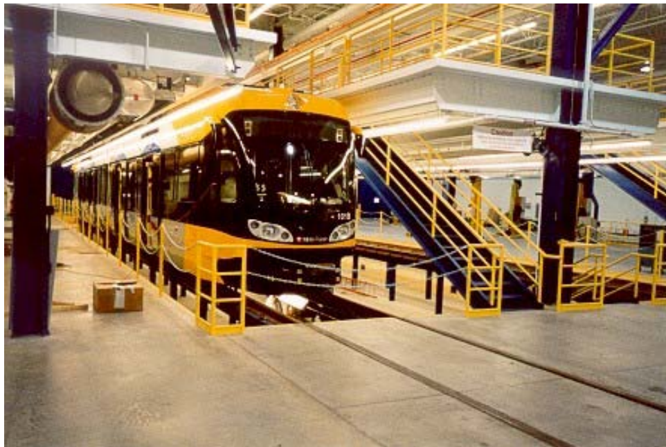
Hiawatha LRT Maintenance Facility, Minneapolis, Minnesota (Photo by Thatcher Imboden, April 2003, http://www.lightrail.com/photos/minneapolis/minneapolis.htm )
