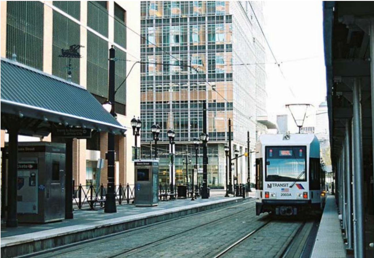
FIG 32. Major new development has been stimulated in nearby Jersey City by the new Hudson Bergen Light Rail Transit line. This suggests considerable potential for light rail-related development on Manhattan's West Side. (Photo by Alexis L. Goldman)
