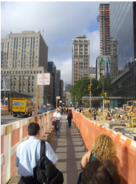
Figure 7 - New York: Transparent Construction Fencing Protecting Continuous Pedestrian Right-of-Way
